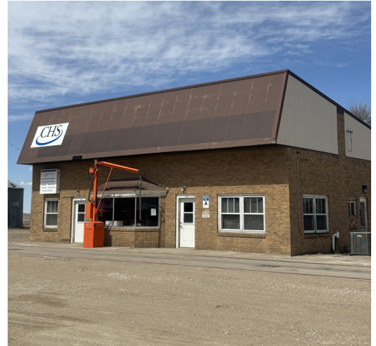
Dallas East Office
